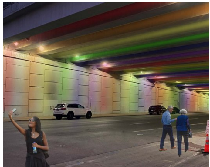
I-65 Underpass Lighting Program
