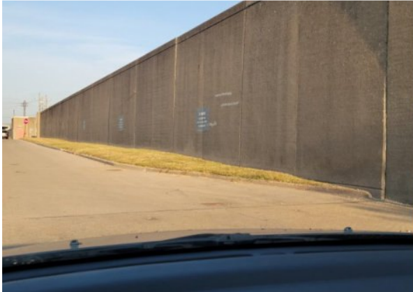
Existing conditions at the Rowan Street flood wall
