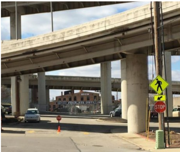
Existing conditions at 9th/Washington Street parking lot
